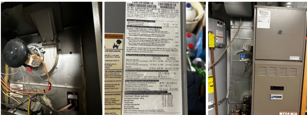
Newly installed induction fan
